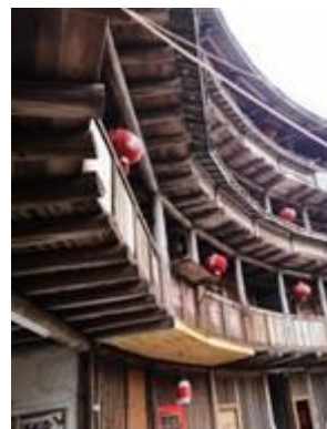
Figure 12: Yude Building, Taxia Village, Shuyang Town
