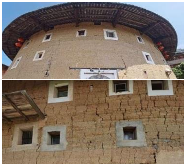
Figure 9: Cave windows of Tianluokeng Tulou
