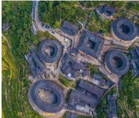
Figure 4: Overhead view of Tianluokeng Tulou
